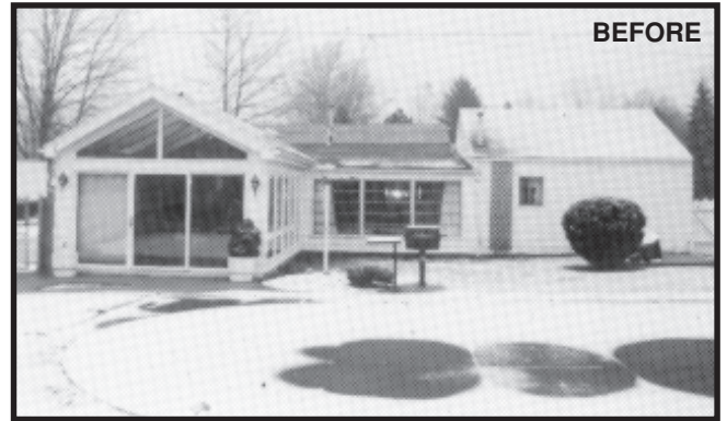
BEFORE: Exterior Flat Roof
