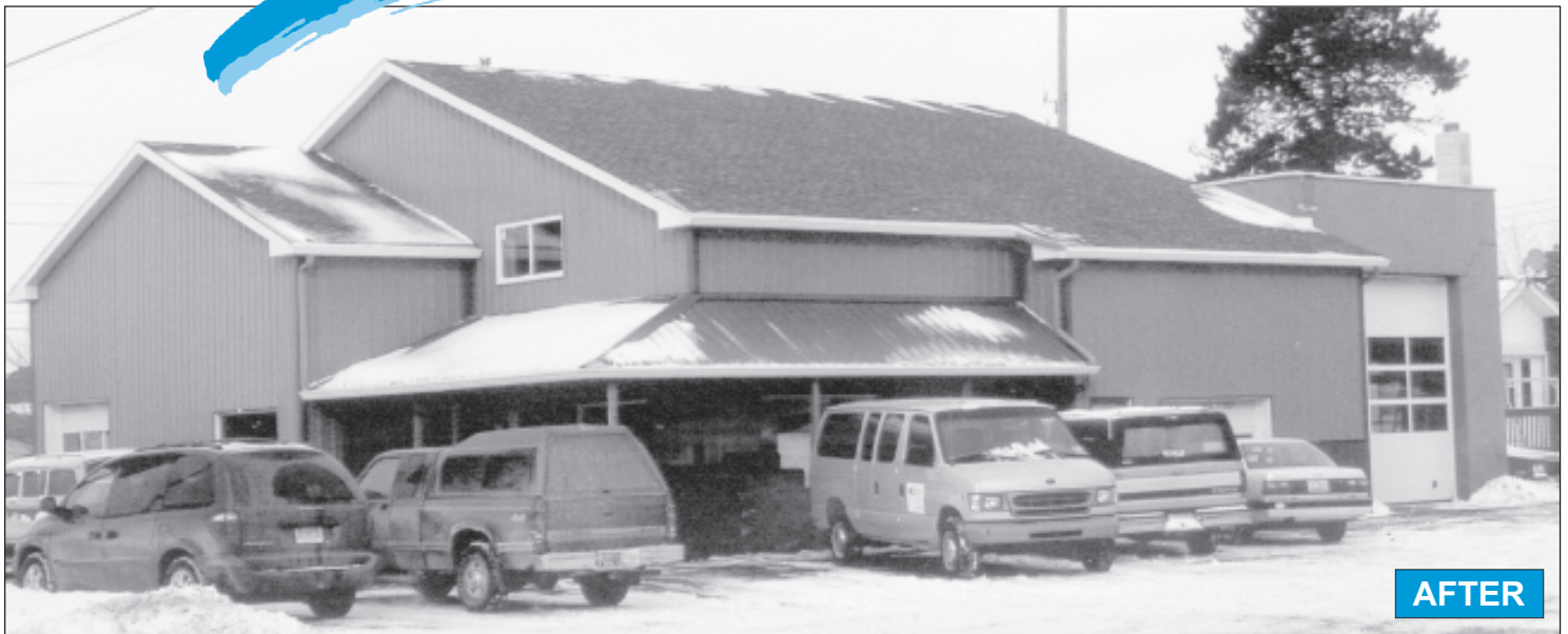
New Gable Roof With Dimensional Shingle
