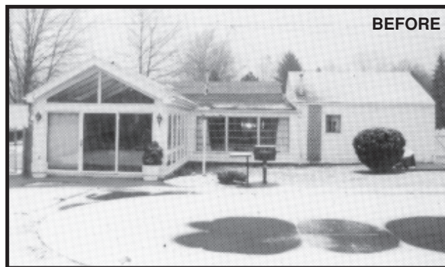
BEFORE: Exterior Flat Roof
