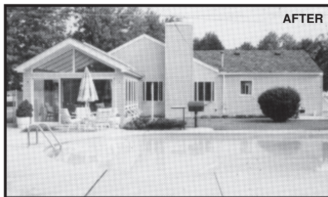
AFTER: New Roof System Offers Better Water Drainage and Updates Appearance Of The Home
