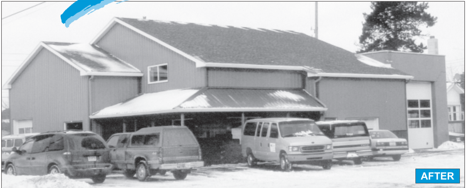
New Gable Roof With Dimensional Shingle
