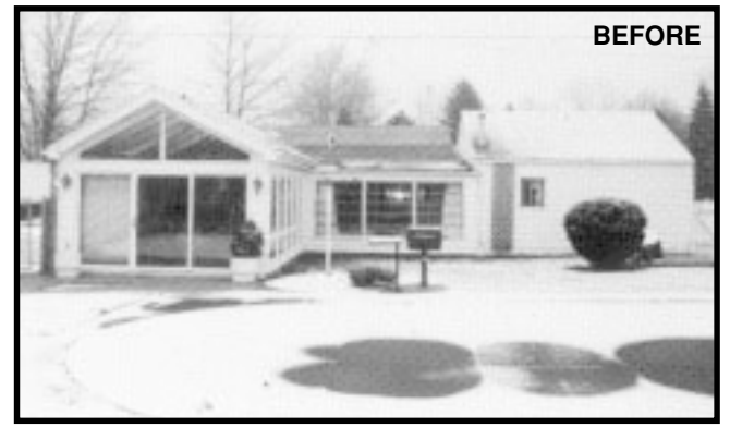
BEFORE: Exterior Flat Roof
