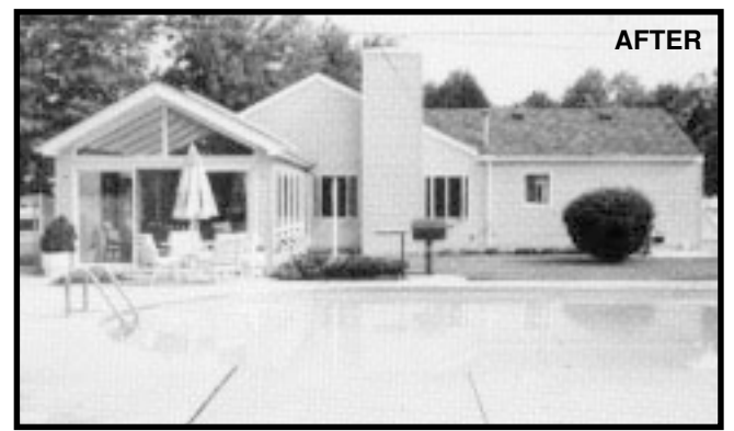
AFTER: New Roof System Offers Better Water Drainage and Updates Appearance Of The Home
